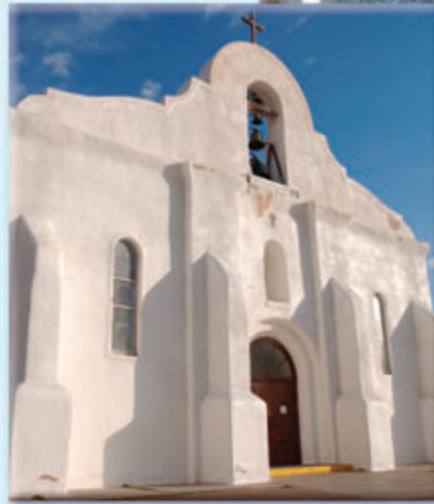
▲ La Capilla de San Elceario San Elceario Mission, near El Paso, is a fine example of Spanish mission architecture in Texas.
